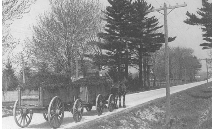
Lakeshore Road was one of the first highways constructed in 1914-22, of concrete in the country. Public protests resulted in Lakeshore Road being re-routed south along Southdown Road (formerly 5 th Line) rather than slicing diagonally through south Clarkson.
