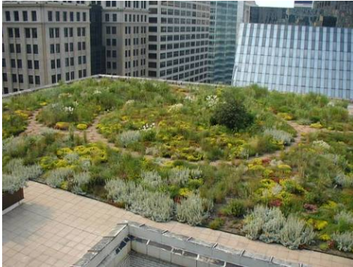
Green Roofs ameliorate the urban heat island effect and support natural habitat.
